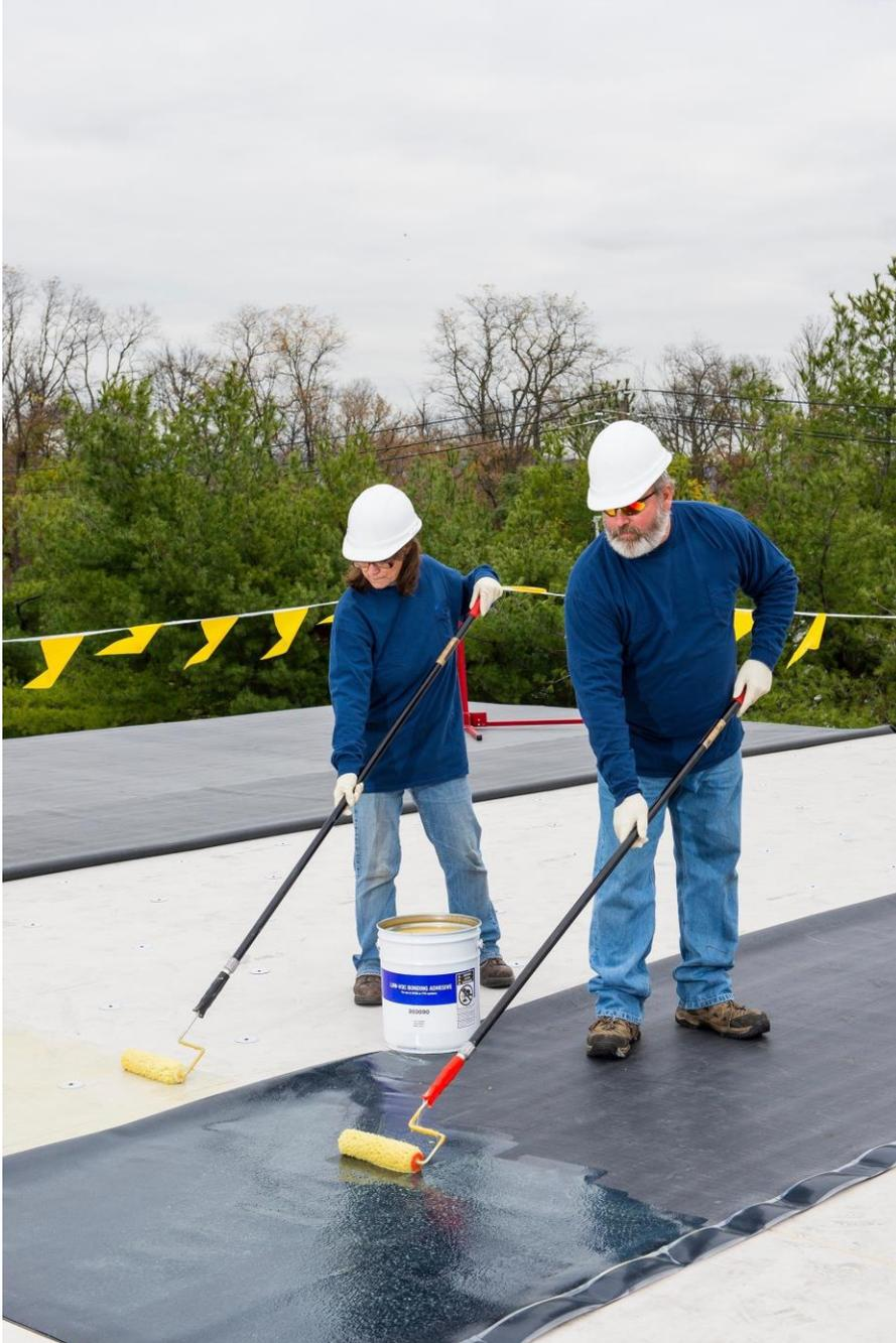
Low-VOC adhesive for installing non-reinforced EPDM roofing membranes
